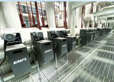
Design+supply of mechanical rapping system of Xiangyang Waste Incineration Plant, Hubei
