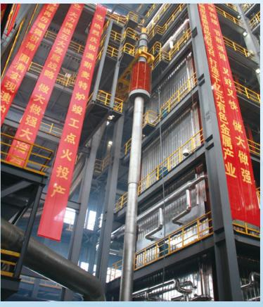
EPC of Ausmelt furnace WHB of Daye Non-ferrous Metals Group
